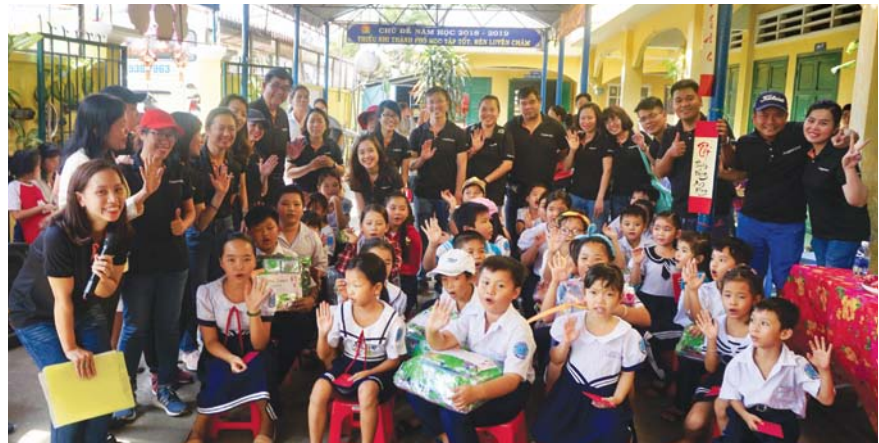
Minor renovation works were carried out by Mapletree staff from the Vietnam office at a primary school where students were from low income families in HCMC, Vietnam
